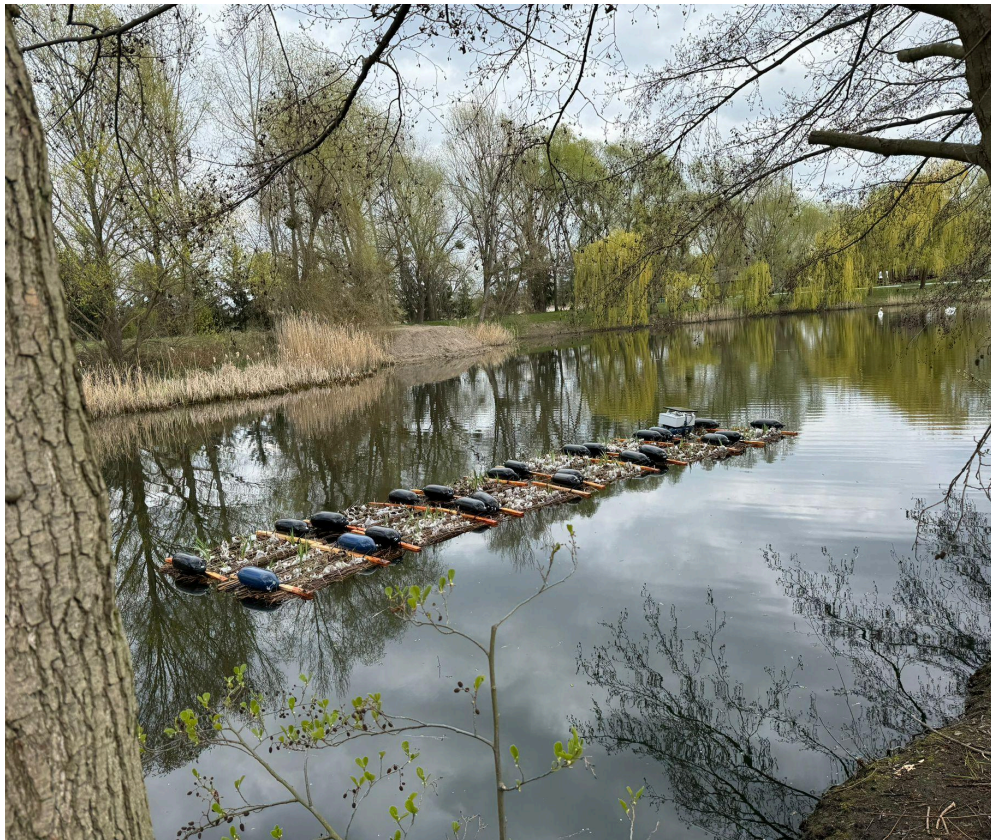
Fig. 11. Twelve launched plant filter islands (source: H2O SCITECH)
