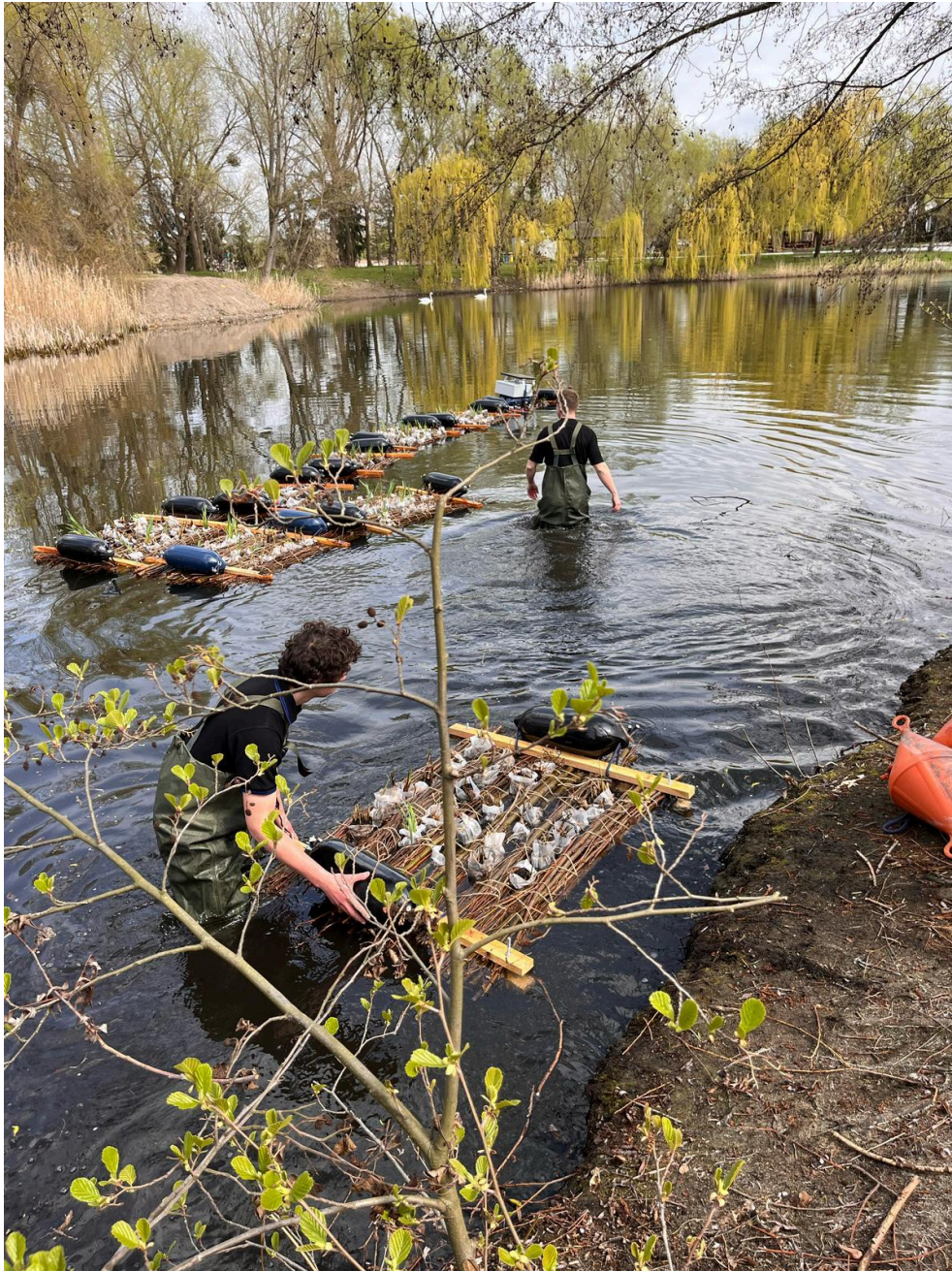
Fig. 10. Process of launching and connecting the islands (source: H2O SCITECH)
