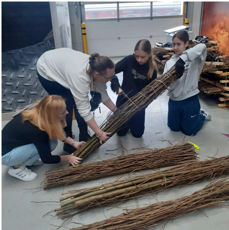
Fig. 4. Preparation of willow fascine (source: H2O SCITECH)
